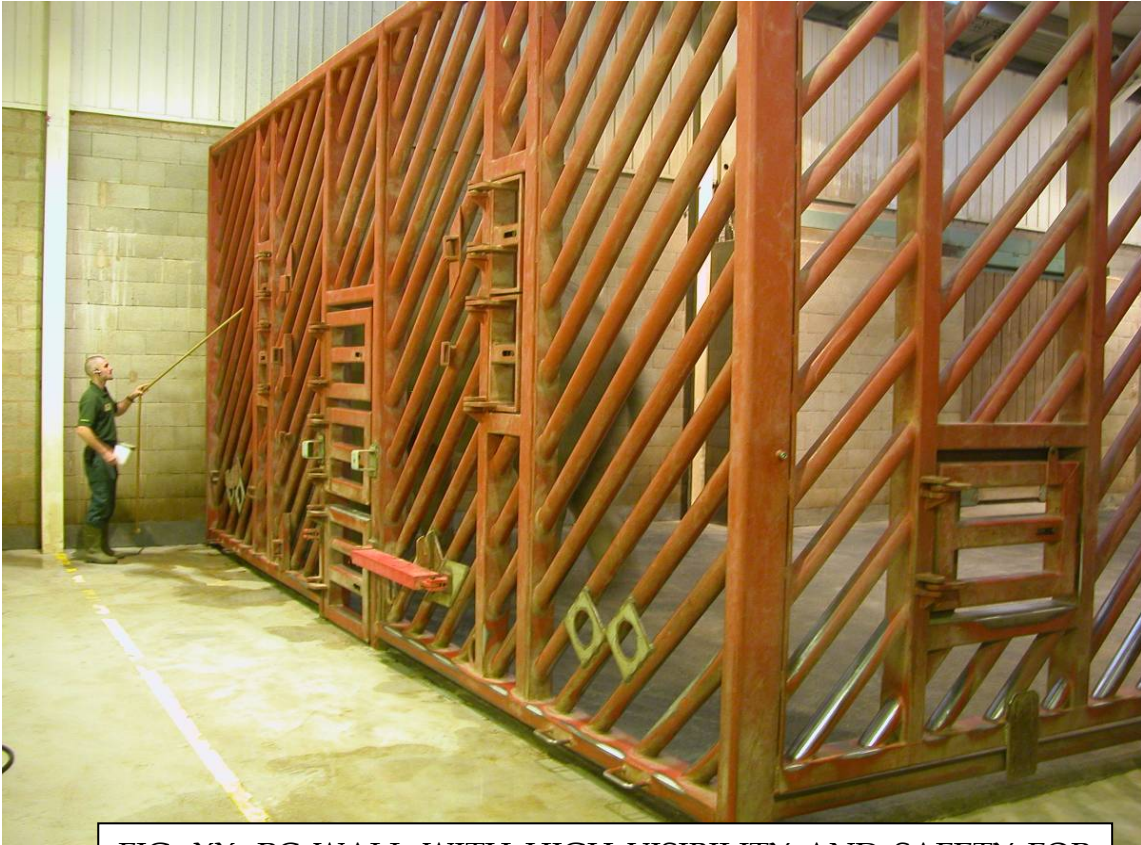
FIG. XX: PC WALL WITH HIGH VISIBILITY AND SAFETY FOR BOTH KEEPER AND ELEPHANT (CHESTER ZOO)
